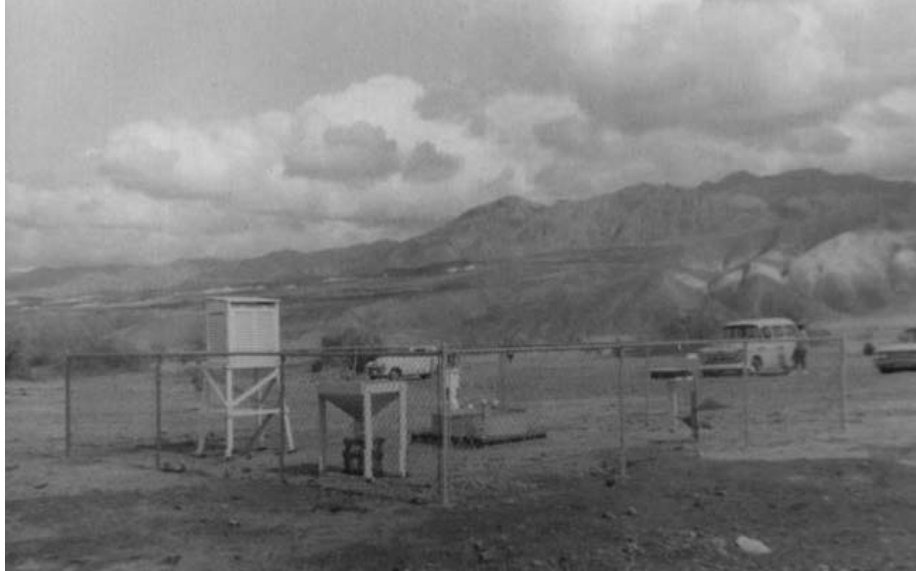
View of the weather station at the Visitor Center at Furnace Creek looking towards the Funeral Mountains. The instrument shelter, evaporation pan and rain gauge can all be seen in this photograph. Photo taken on February 20, 1962. Photo Credit: NWS Las Vegas archives.
