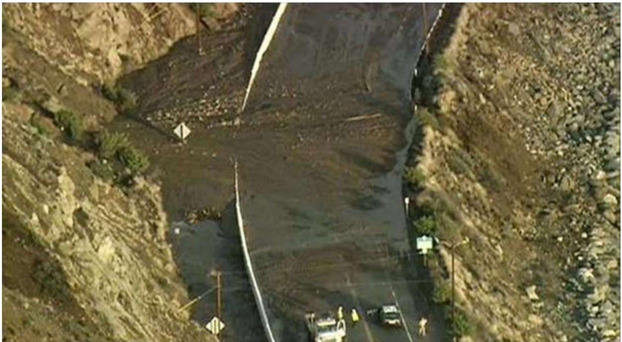
Fig. 22. Image from 12 December 2014 showing an area of the Pacific Coast Highway (PCH) just north of Deer Creek Road that was inundated with mud and rocks following flash flooding and debris flows. Image is courtesy of NBC.
