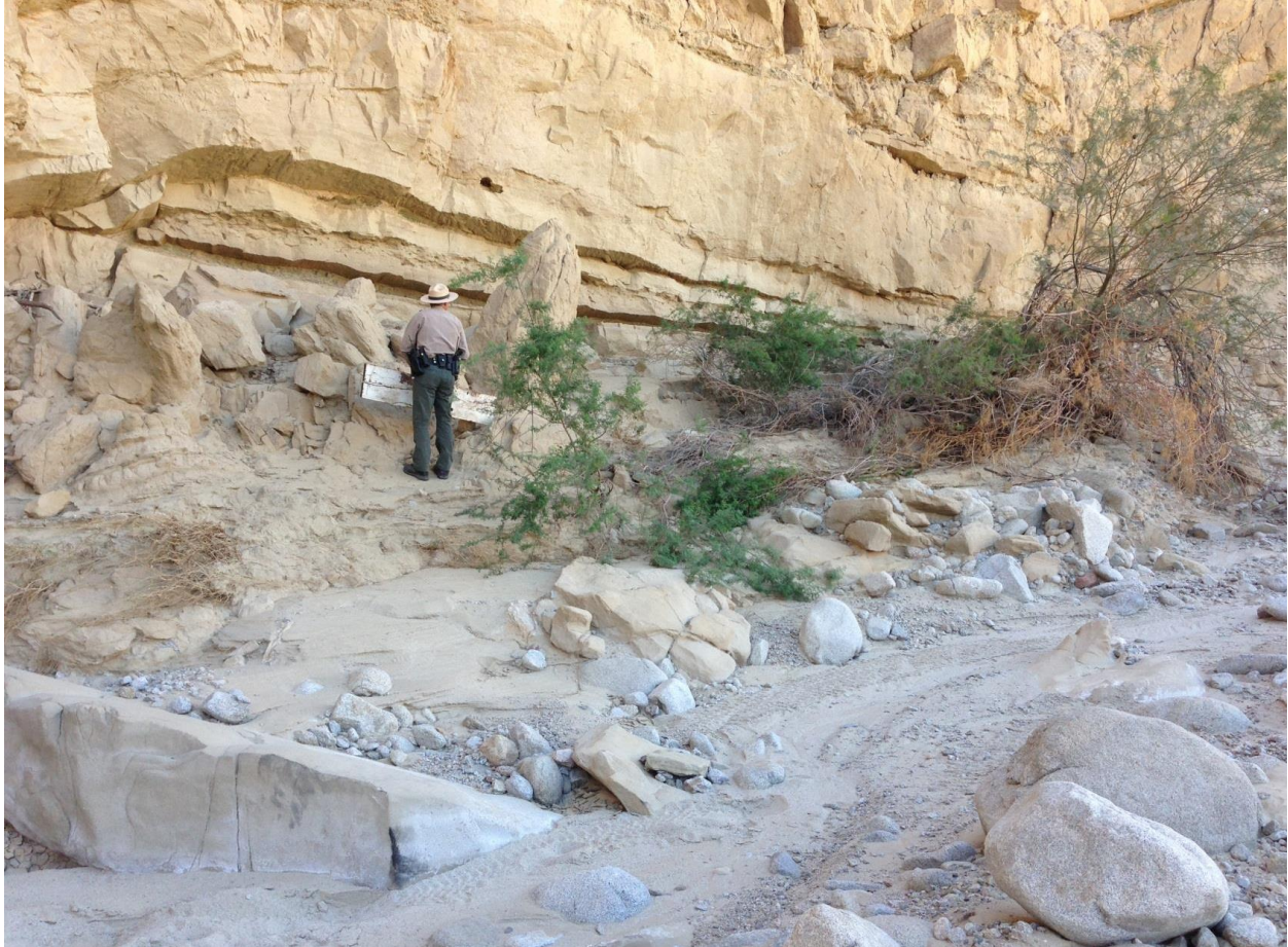
Figure 3. Looking at high water marks along North Fork of Fish Creek. Wood debris found wedged 15-feet above channel floor. This debris was noted not to have been there prior to the flood. California State Parks ranger Steve Bier is in the picture. Photo Credit: NWS San Diego.
