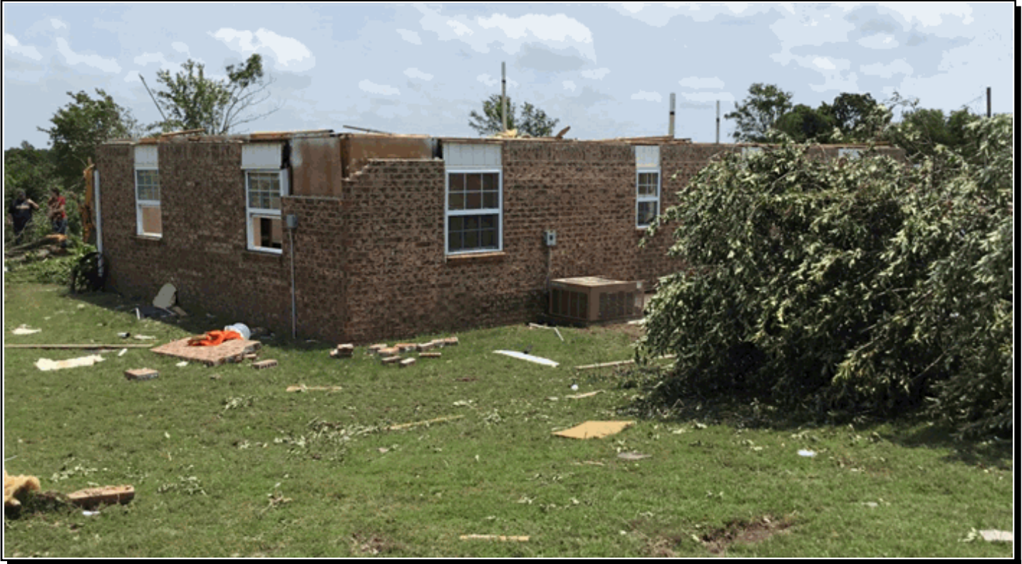
An EF-2 tornado destroyed several mobile homes, severely damaged permanent homes, and snapped or uprooted numerous trees in a wide and lengthy path from near Jay, Oklahoma to north of Southwest City, Missouri, on the evening of May 22, 2019. Photo by Ed Calianese, WCM, NWS Tulsa Oklahoma.
