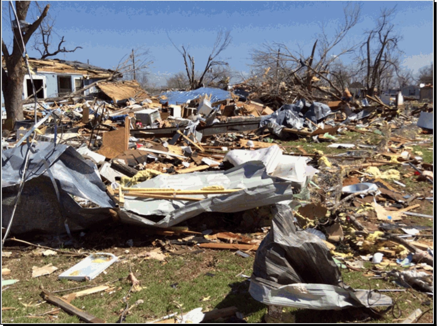
An EF-2 tornado destroyed 58 mobile homes and severely damaged two permanent homes in the River Oaks Estates Mobile Home Park in Sand Springs, Oklahoma, on the evening of March 25, 2015. One fatality and 30 injuries resulted from this tornado. Photo by Ed Calianese, WCM, NWS Tulsa Oklahoma.
