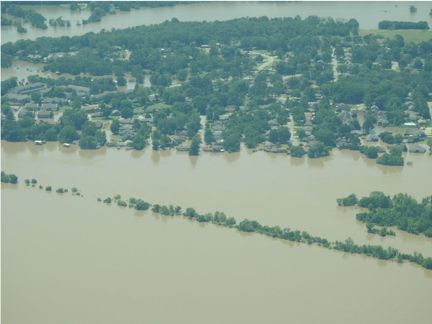
Image D. View of the Arkansas River at its crest on May 31, 2019 flooding a neighborhood in Fort Smith, AR, looking south. Photo credit: Steve Piltz
