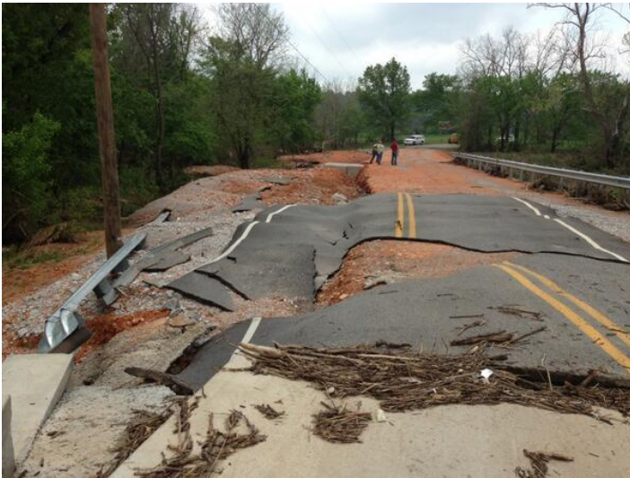
Figs. 12. Asphalt removed off of S. Opal Road in Benton Co. by high water. Photo courtesy of Benton Co. EM Robert McGowen. 5/10/2013
