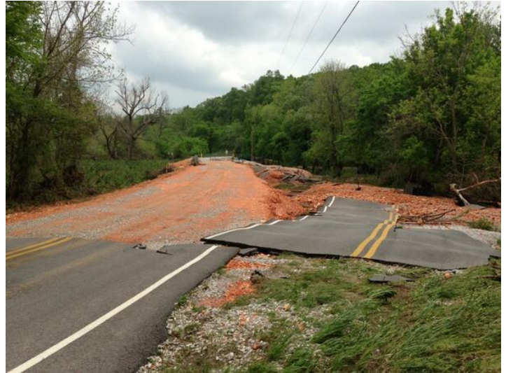
Figs. 12. Asphalt removed off of S. Opal Road in Benton Co. by high water. Photo courtesy of Benton Co. EM Robert McGowen. 5/10/2013
