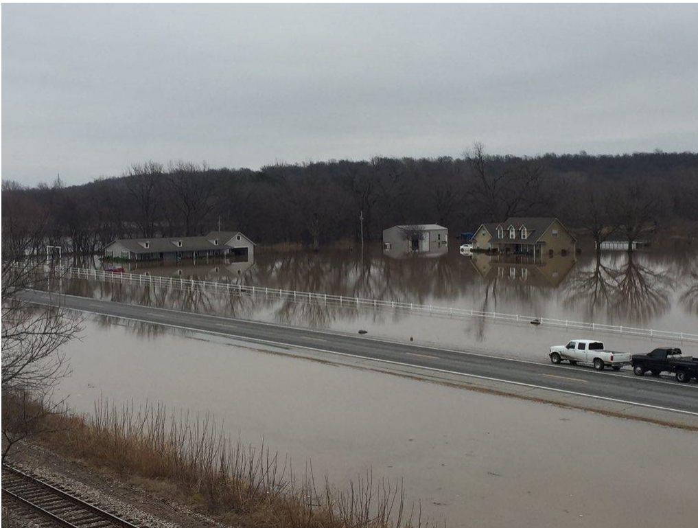
Fig. 38. Muskegee County flooding on Dec. 29, 2015. Image: Von Castor
