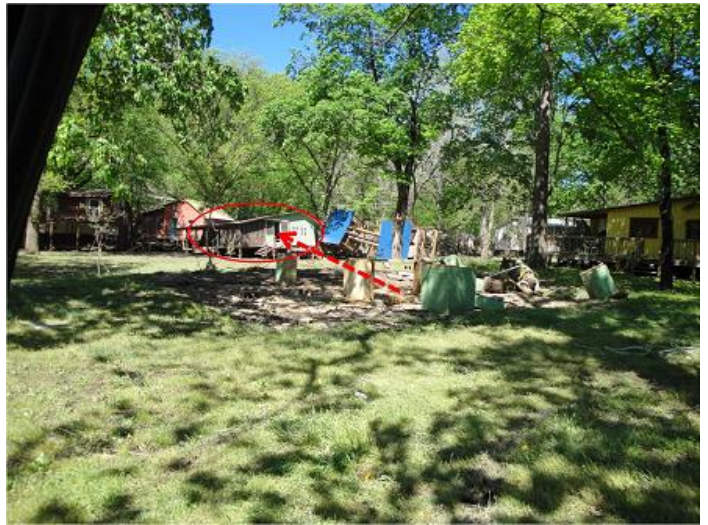
Fig. 16. Fiddlers Bend along the Illinois River. Green home was washed from its foundation. Red home was also moved off its foundation.
