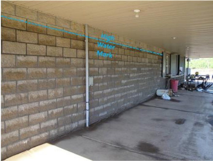
Fig. 15. Flooded business along the Illinois River near Watts. Water reached approximately the blue dashed line.
