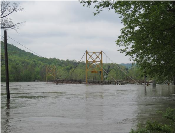
Fig. 17. Suspension bridge on Hwy 187 over the White River.
