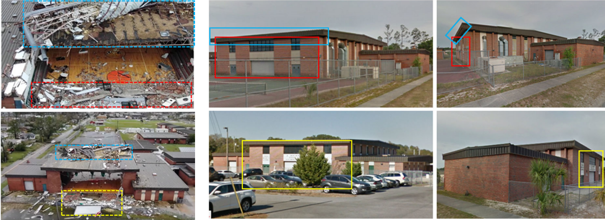
(a) After hurricane Michael
