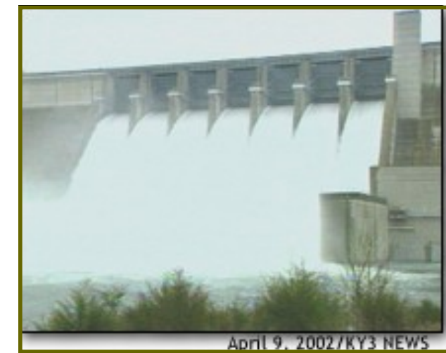
Spillway gates open to relieve lake levels after heavy rains.
