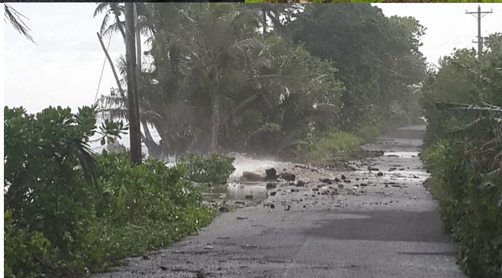
Damaged roads in Kosrae
