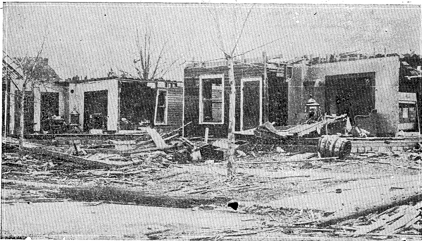
Griffin, Ind., showing how walls of some of the houses were blown out by explosive force, leaving articles of furniture in position on the room floors.
