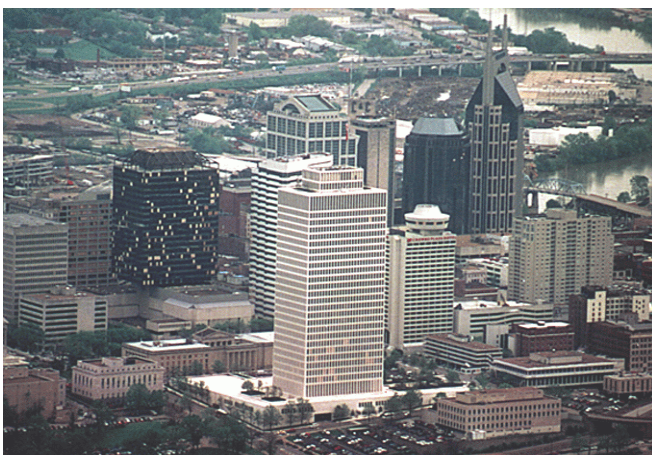
(Photo courtesy of Tim Marshall, Structural Engineer, Haag Engineering, Dallas, TX)
