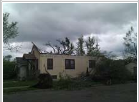
Home damage in Minneapolis, MN
