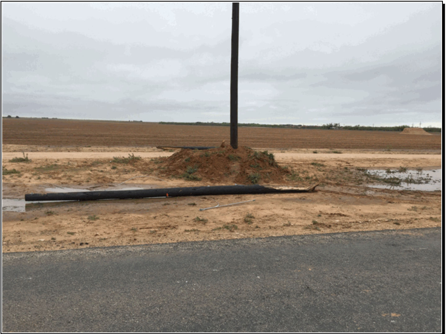
A thunderstorm produced wind damage near Elbow, Texas. Telephone poles were snapped due to the strong winds. Photo courtesy of Mark Strobin.
