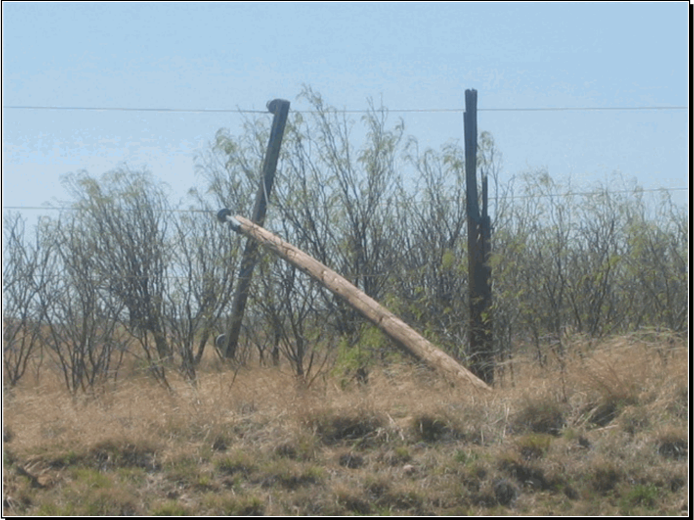
A power pole was snapped near its base as the tornado passed near its location. This photo was taken by Pat Vesper, WCM Midland WFO, during the damage survey.
