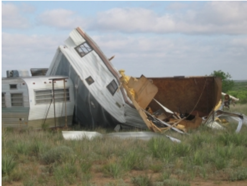
Eight mobile homes were destroyed just before the tornado dissipated twenty miles southeast of Colorado City. The trailers served as bunks for hunters and gamers visiting the ranch property, and were not occupied at the time of the storm. The above photo shows one of the trailers as it came to rest against a small camper trailer.
