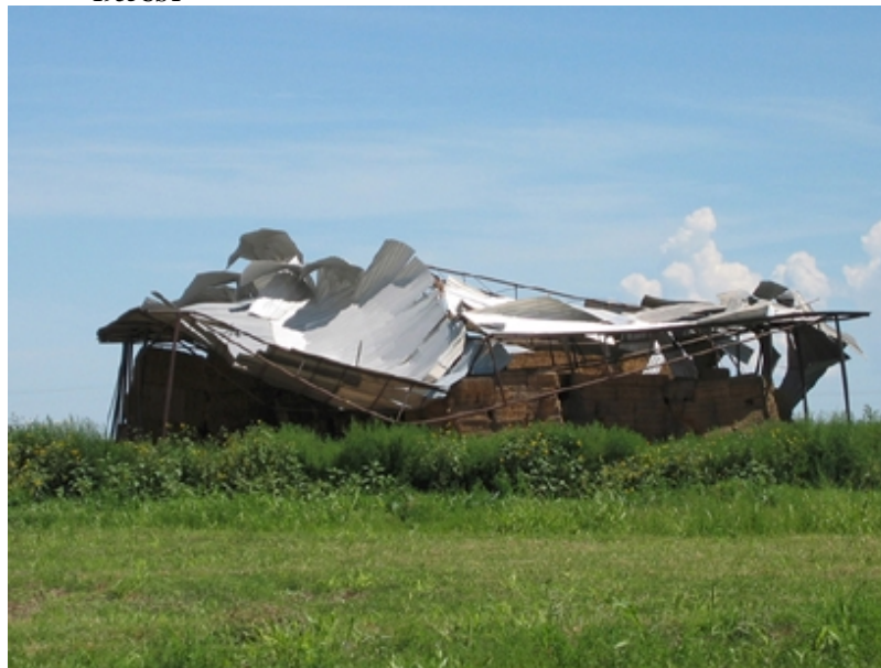
Two large hay barns were destroyed as a tornadic supercell tracked south across central Pecos County. A National Weather Service damage assessment team determined the damage was the result of severe rear flank downdraft winds on the back side of the storm. Photo courtesy: National Weather Service, Midland/Odessa, Texas.
