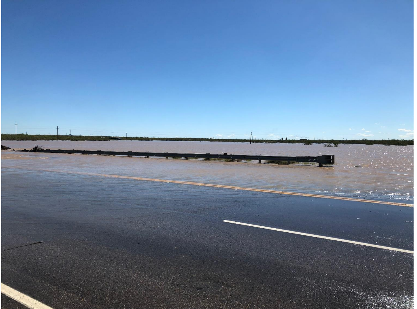
Figure 10 – Flooding along TX 158 between Midland and Garden City, Texas.
