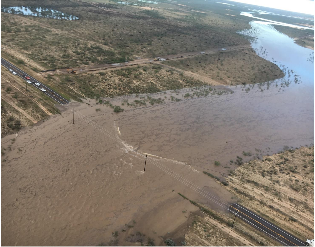
Figure 6 – Helicopter view of Flooding on TX 137 near the Intersection of TX 158.
