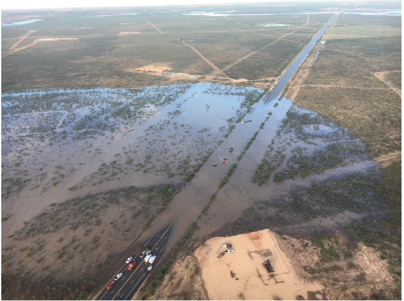
Figure 7 – Helicopter view of Flooding on TX 158.
