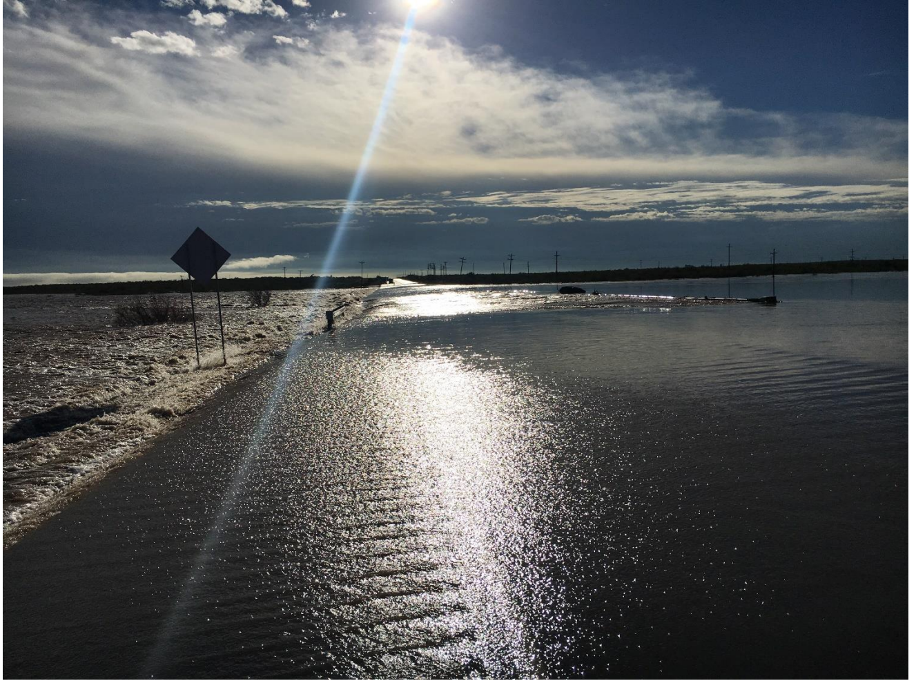
Figure 8 – Flooding along TX 158 between Midland and Garden City, Texas.
