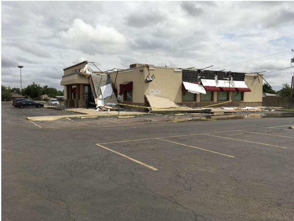
Figure 12 – Roof damage at a restaurant near TX-158 BR and W Louisiana Ave in Midland, Texas.
