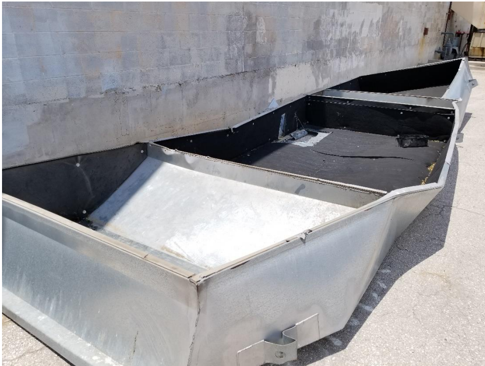
Figure 6 – Pieces of HVAC equipment at Albertsons in Hobbs, New Mexico.
