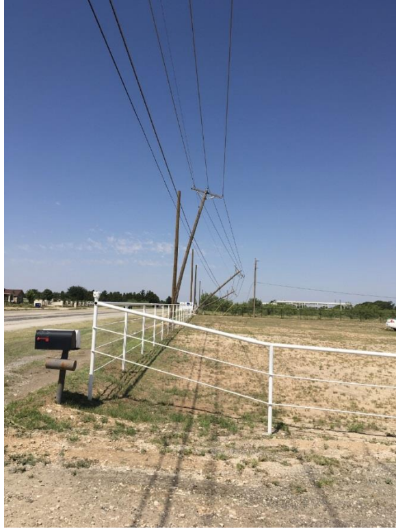
Figure 6 – Power polls snapped along W 16 th Street in West Odessa, Texas.
