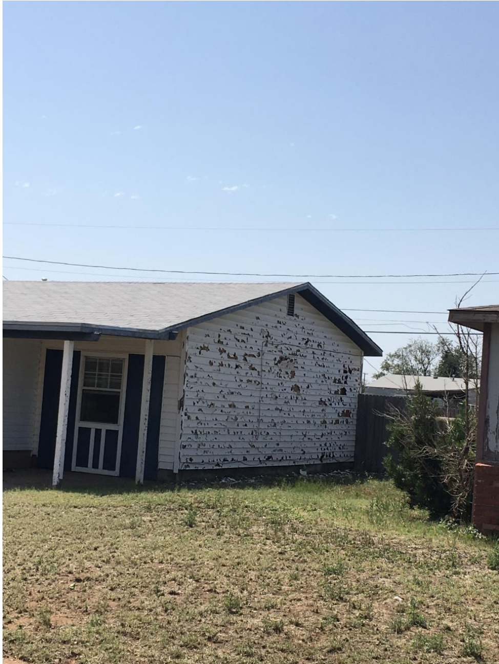
Figure 12 – Hail damage to a house near E 42 nd Street in central Odessa, Texas.
