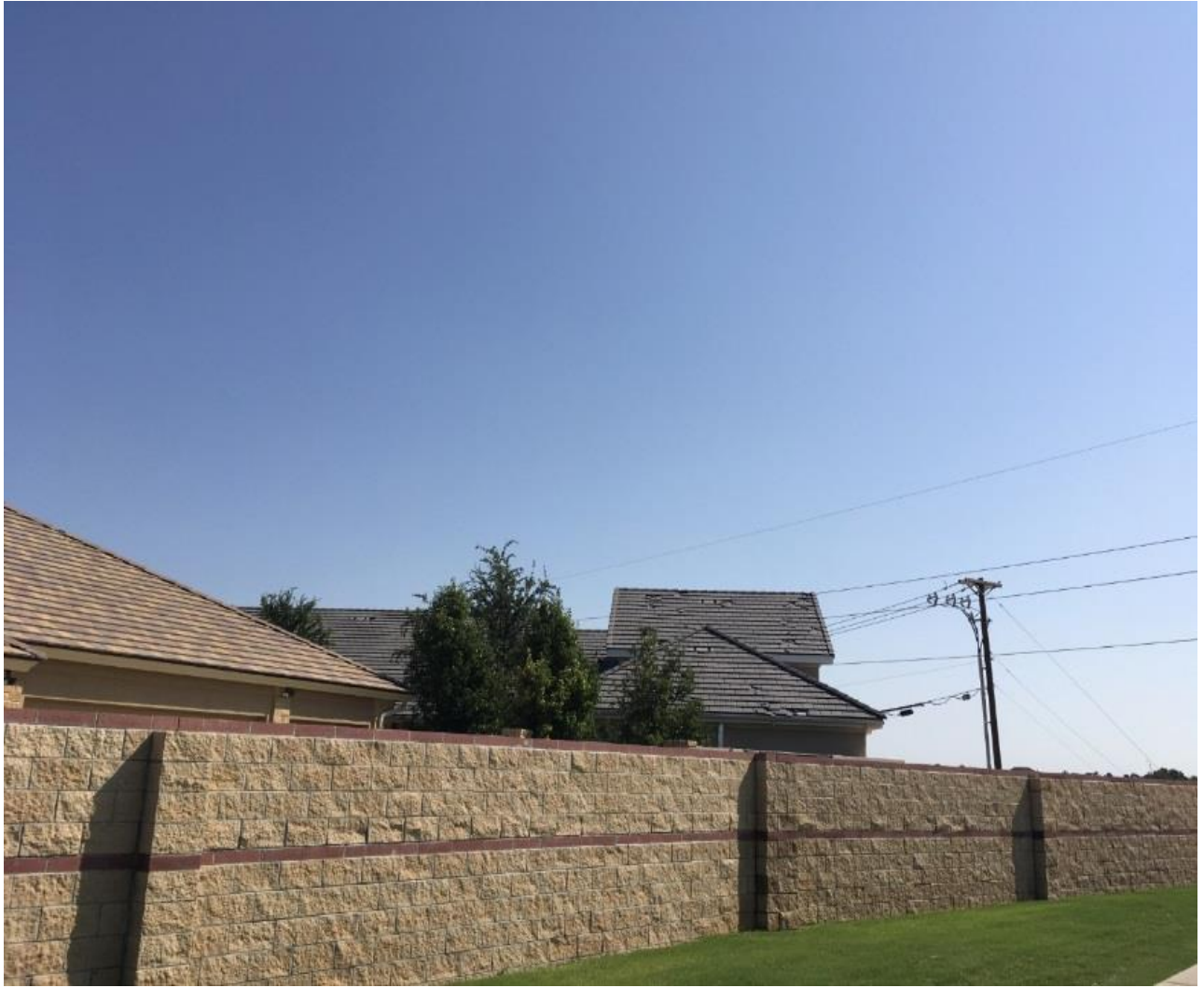
Figure 10 – Roof damage from hail at the Odessa Country Club in Odessa, Texas.
