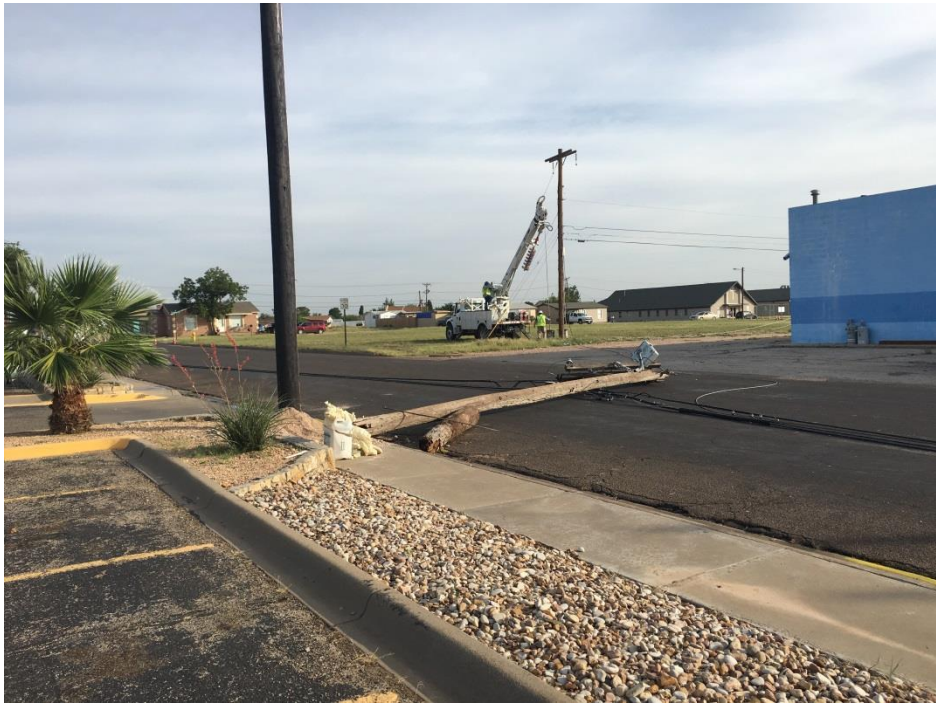
Figure 5 – Power poles snapped at the corner of Wall St and Powell St (Courtesy of Amber Hluchan).
