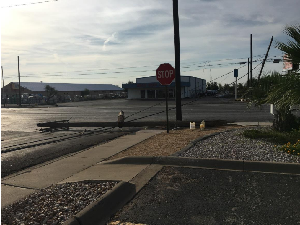
Figure 4 – Power poles snapped at the corner of Wall St and Powell St (Courtesy of Amber Hluchan) .
