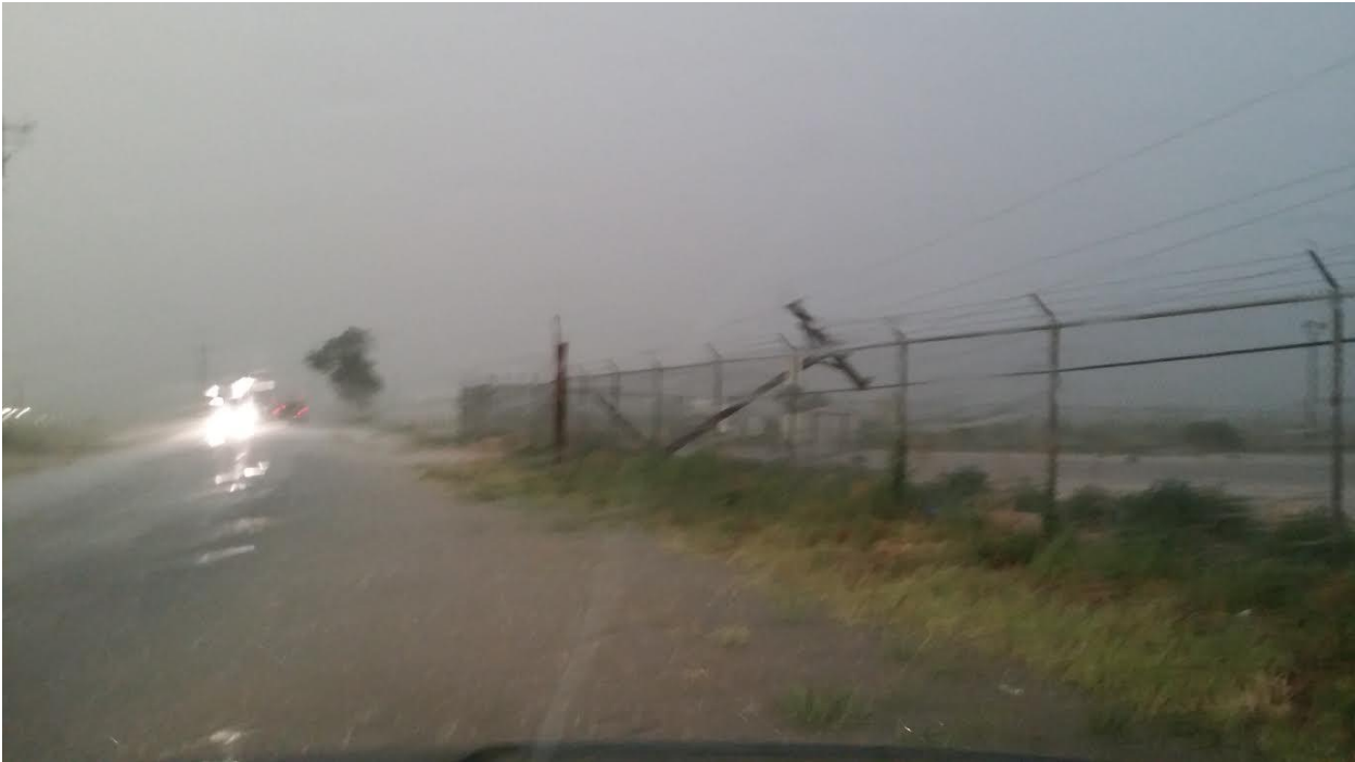
Figure 8: Snapped power poles in northeast Midland (courtesy of Chris Dewrell).
