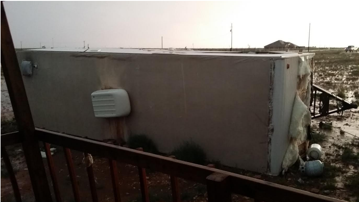
Figure 6: Overturned travel trailer in northeast Midland (courtesy of Chris Dewrell).
