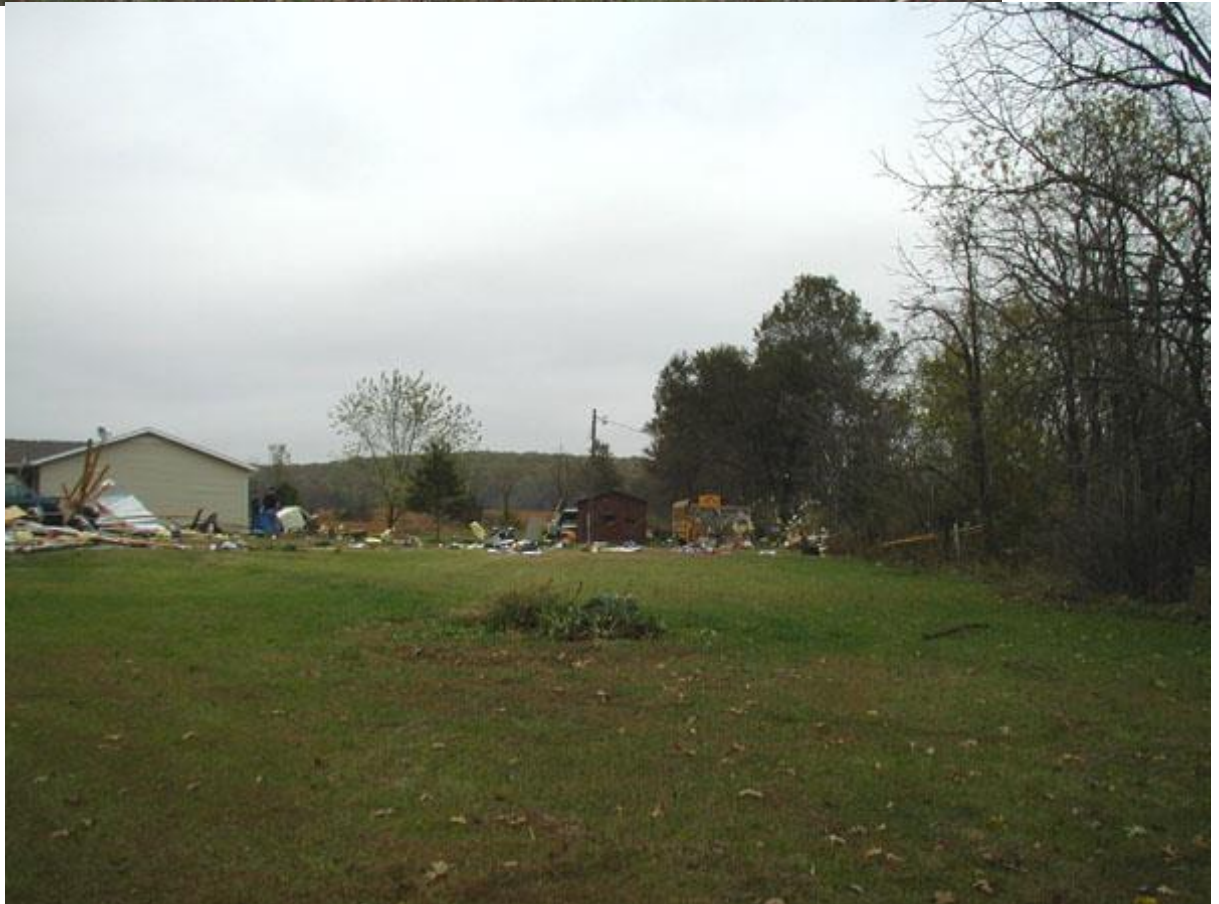
North facing view of the destroyed garage and debris field along the east side of County Road 219 northeast of Fredericktown. Note the single story home which is just north of the garage was completely untouched by the tornado.
