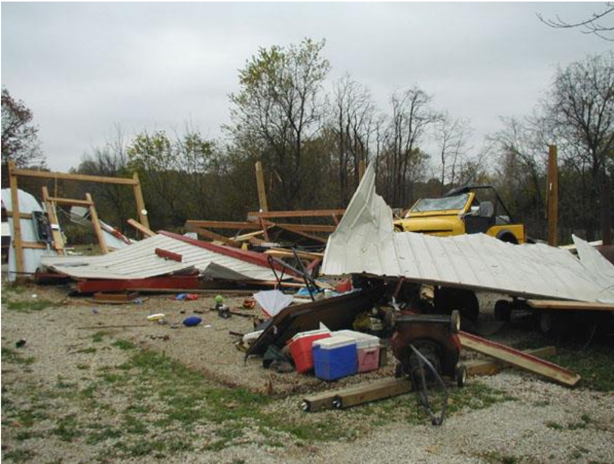
Destroyed minimally-anchored and unattached garage along east side of County Road 219 northeast of Fredericktown. Strewn debris from the garage is shown in the previous picture.
