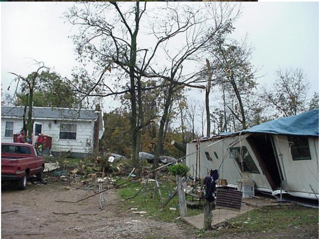
Damage to a house trailer, and home along the east side of East State Highway (one mile northeast of Potosi Missouri) from the second of five tornadoes. Viewing southeast.
