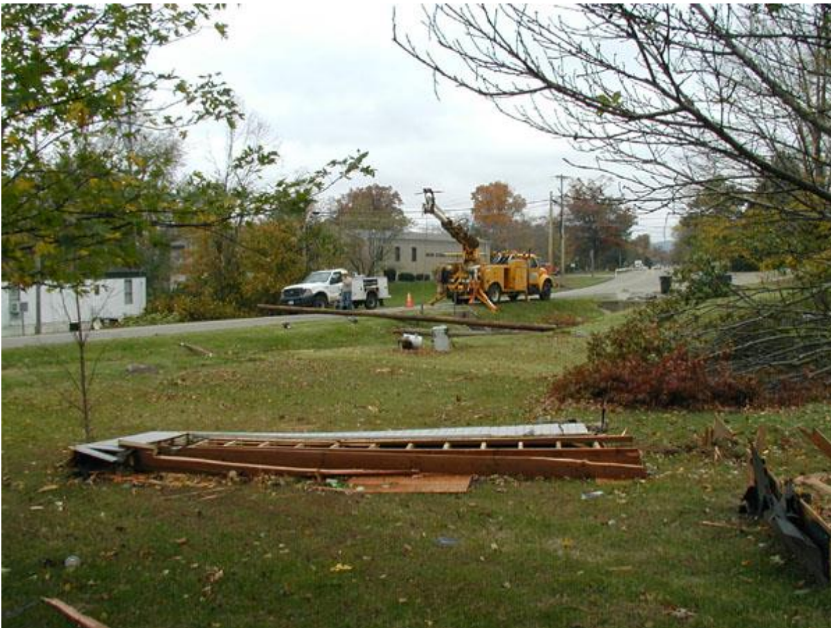
Iron County Health Center in rear center of picture behind the yellow utility company truck. A portion of the Health Center roof carried some 75 yards to the northeast in the lower center of the picture along with missiles in the lower right corner.
