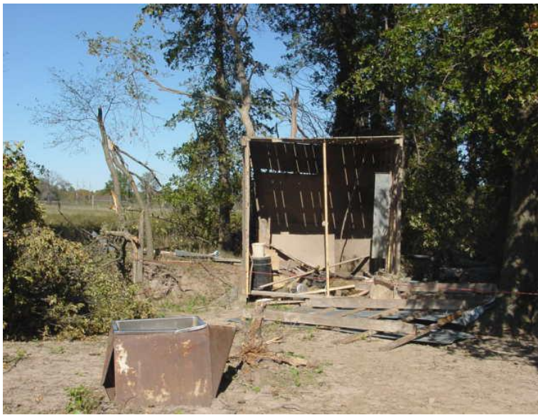
Horse stable severely damaged by the weak tornado near County Road 264 (Callaway County). Parts of the horse stable were tossed 30 to 40 yards to the north-northwest.
