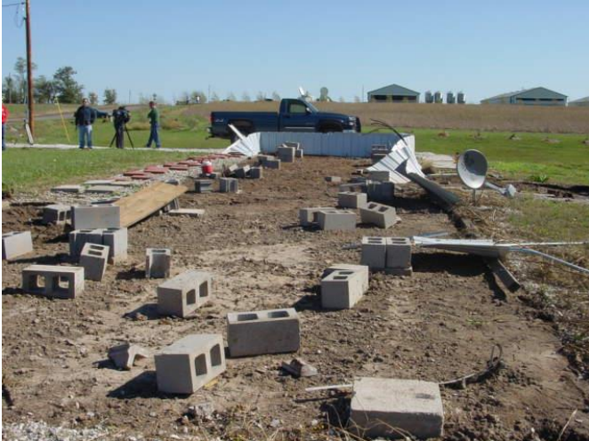
(Tornado #2 - northwest of Paris, MO) A few remains of the single wide mobile home just south of Highway F. (Viewing east).
