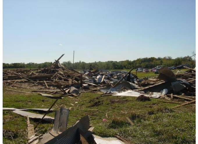
(Tornado #2) Remains of a large barn and machine shed. Debris from this barn and machine shed was noted from the initial touchdown location and spread up to 4 miles north of this site. (Viewing southeast).
