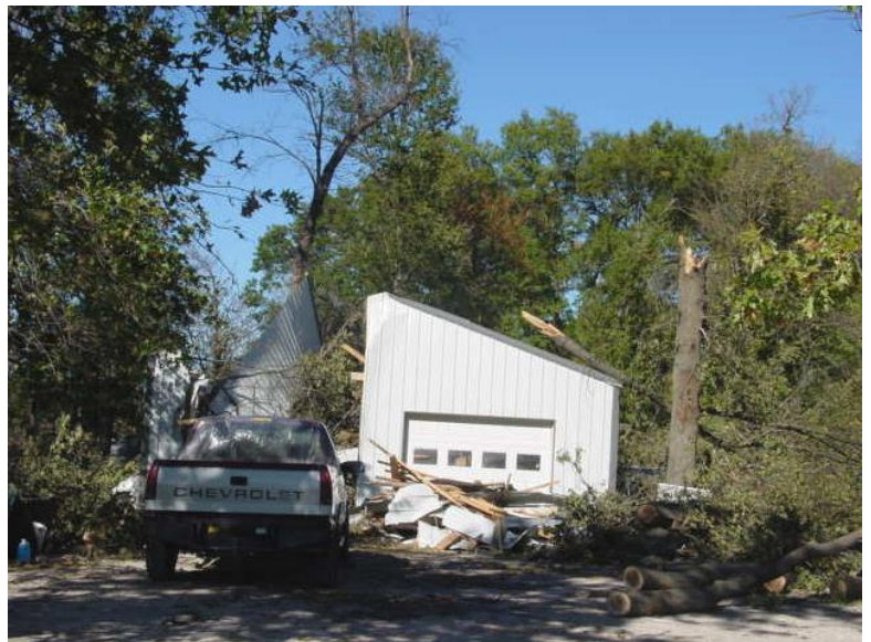
A large garage was severely damaged by the weak tornado near County Road 264 (Callaway County). Parts of the garage were tossed 30 to 40 yards to the northeast. Additional tree damage was found 60 to 80 yards to the northeast. (Viewing north).
