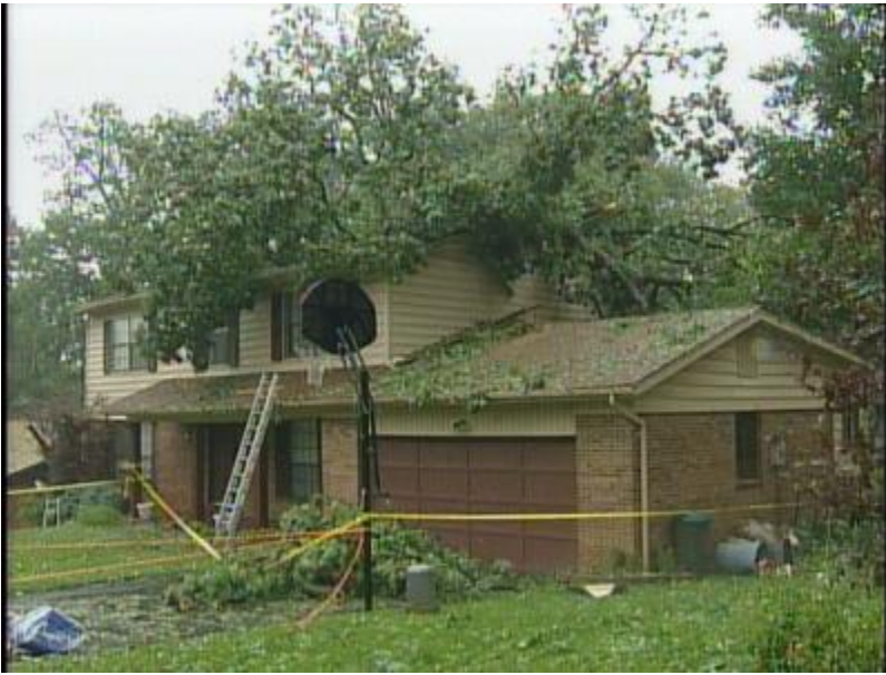
Tree blown down onto a house. Photo courtesy of KSDK Channel 5.
