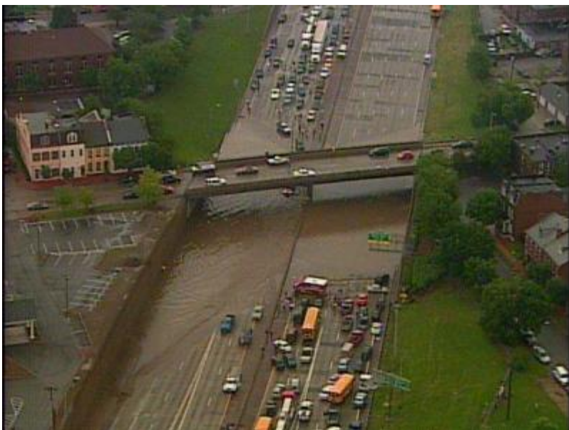
Flooding on I-55. Photo courtesy of KSDK Channel 5.
