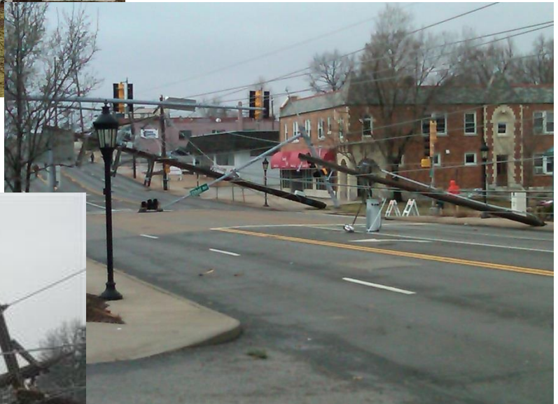
Damage to power poles in Richmond Heights, Missouri. Photo courtesy of Tim Breckinridge.
