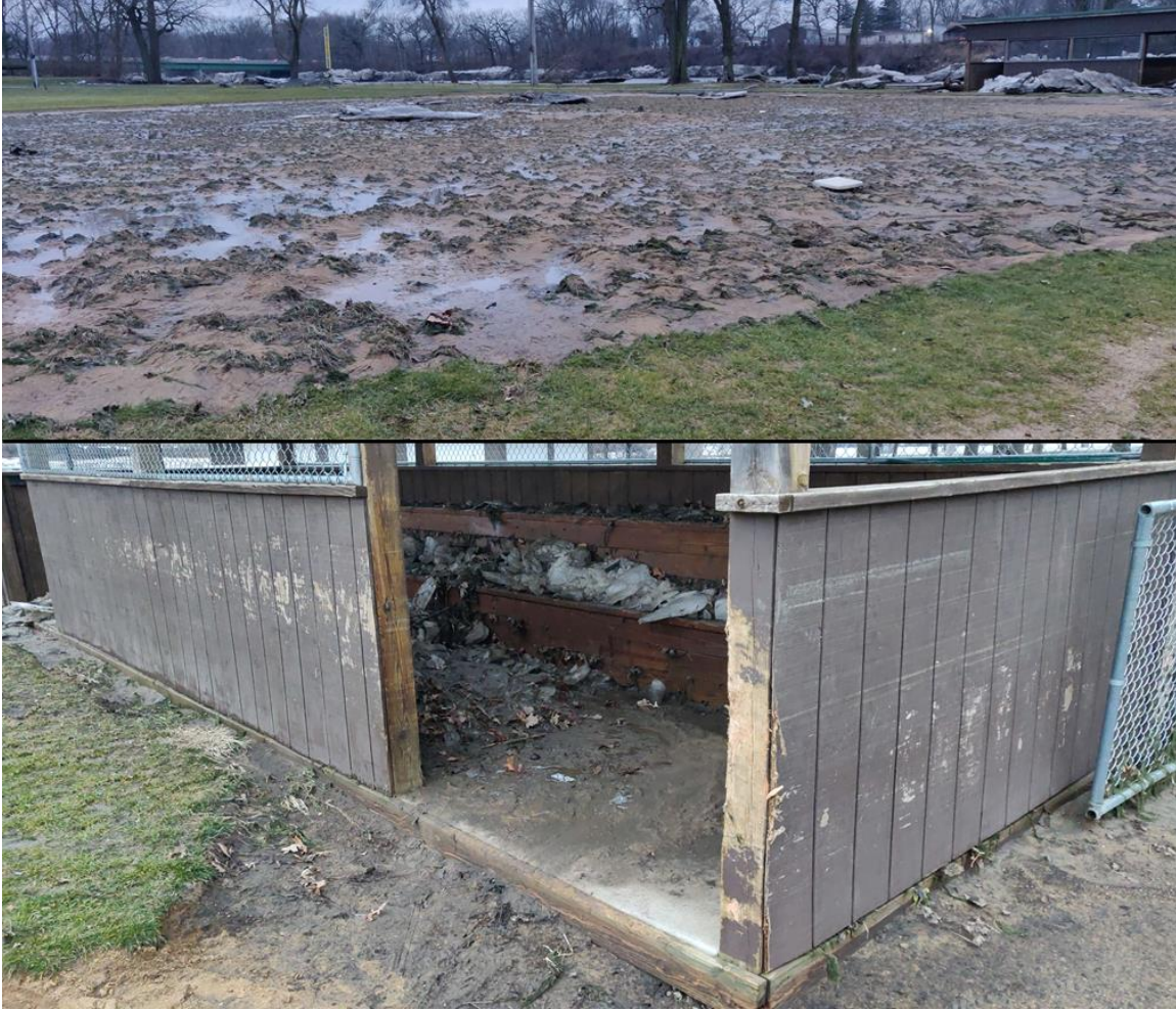
Figure 15. Damage to a baseball field at the North Island Park (downstream end) in Wilmington due to flooding and ice flows. Photographed on January 30.
