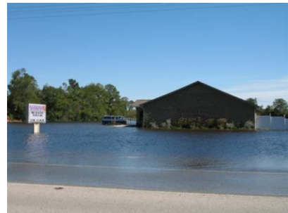
A church along Highway 171 is engulfed by flood waters
