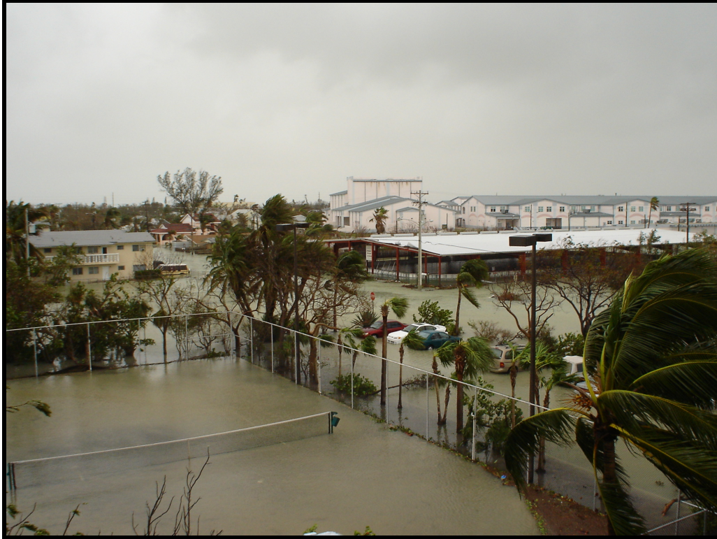
Fig. 10. Storm surge flooding around 1030 EDT, 24 October, Bertha Street and Atlantic Boulevard intersection, Key West, FL (photograph by Chip Kasper)
