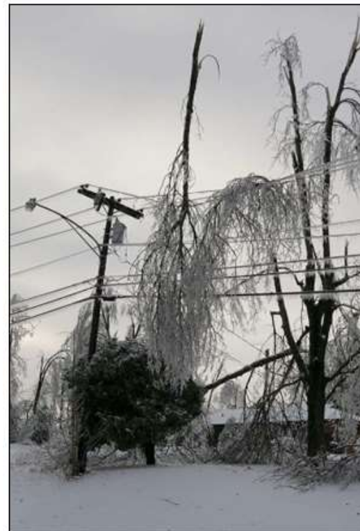
2009 Ice Storm Damage. Photo courtesy NWS Paducah website
