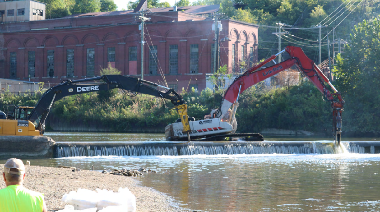
Photo 2: Low head dam removal
