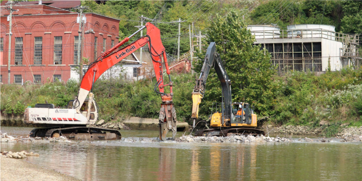
Photo 3: Dam removal almost completed
