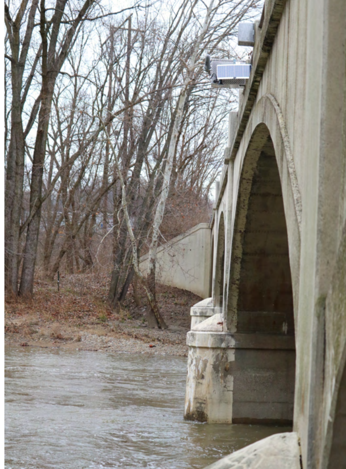
Photo 4: New gauge location on Lafayette Ave bridge
