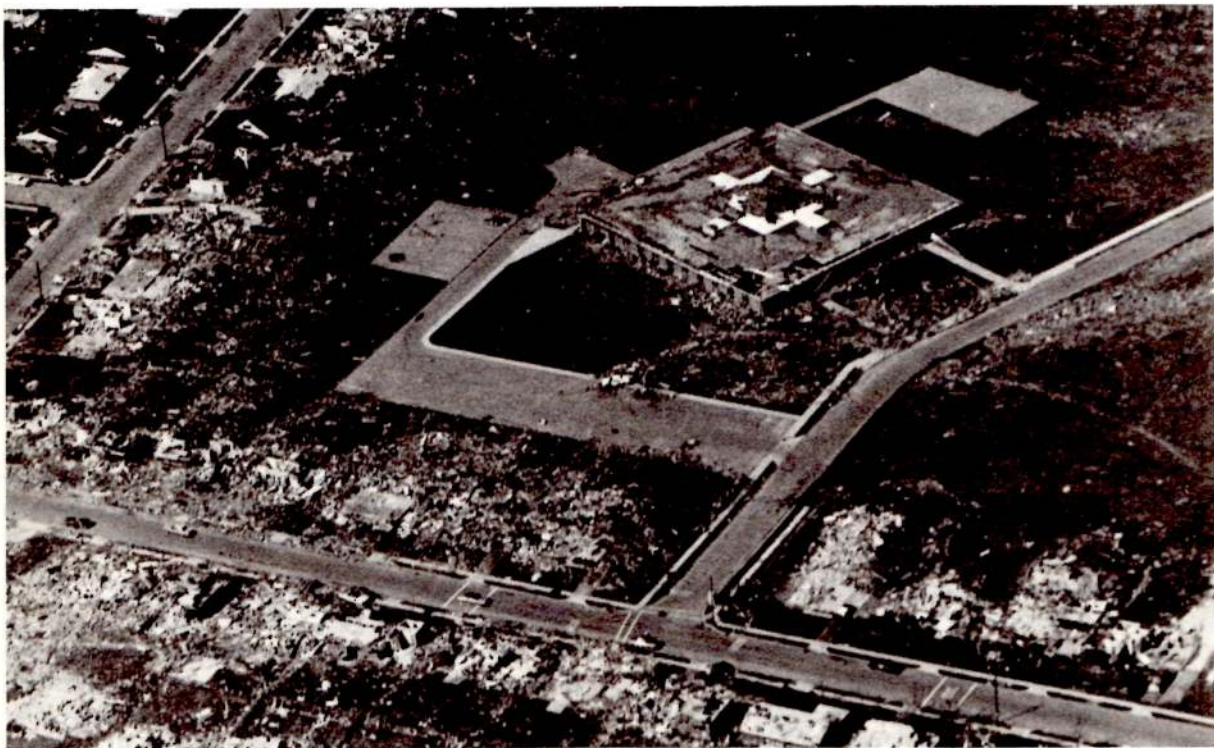
Damage to school and nearby residences.
