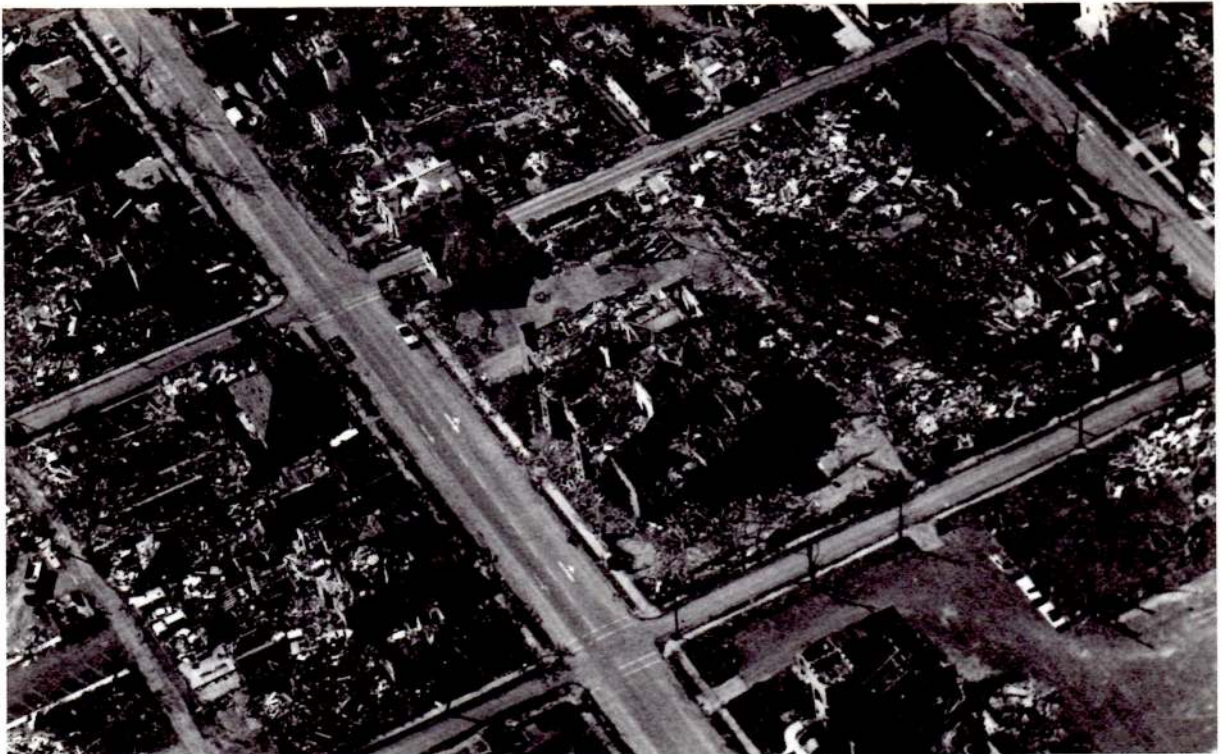
Damage to school and nearby residences.
