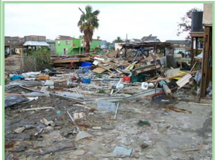
Surge damage in Bayou Vista, Texas due to Ike
