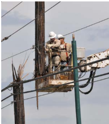
CenterPoint Energy crews repair pole in South Houston, Texas
