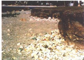
Coastal erosion undermining inland rocks
