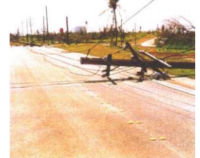
Weakened, unguied wooden power poles can break
