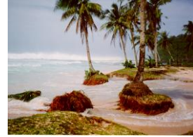
Some near-coastal erosion at high tide
