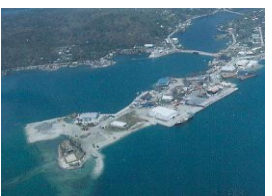
Coastal damage at Yap from Ty Sudal 2003
