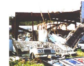
Poorly reinforced hollow-block walls can topple
