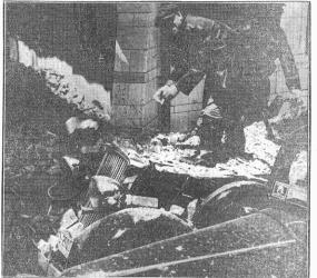
FALLING BUILDING WRECKS AUTO —Parted right where the automobile bullock passed was sitting a few days ago, this automobile was crushed yesterday when the building at 107-109 South Fourteenth street collapsed. The car belongs to Roy Felton, Tenney Ogden's former manager.
