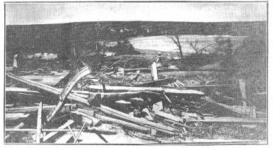
PIONEER HOME DESTROYED BY SOUTHWESTERN NEBRASKA TORNADO —On the site of one of the oldest homesteads in Red Willow county, now occupied by Clifford Blaska, this wreckage shows the havoc wrought by Friday's tornado. The wreckage was an added disaster as cranks and rivets were at flood crest as the tornado hit. Note water-filled stream in background. (All rights.)
