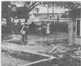
BUILDING A HOME —Shaw here is the arrival of the first tent sent by the Red Cross at McCook to hold a home for a family displaced by the flood. Workers were pulling up the tent yesterday, designed for the Harley Coop family, including three children.
