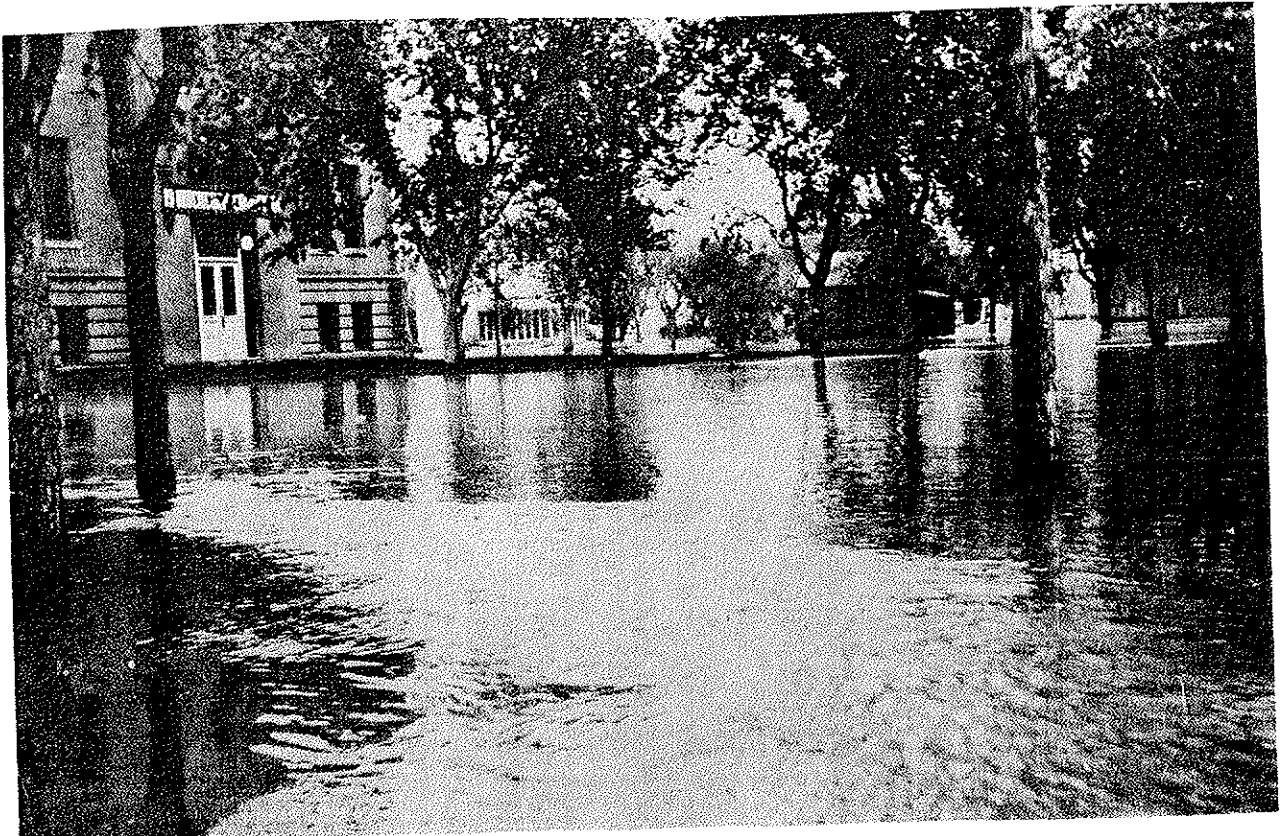
Hitchcock County Courthouse and grounds inundated by 1935 flood
