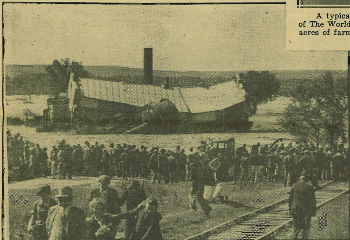
Thirty-six men are marooned today in the McCook, Neb., power plant, shown here. They had fought vainly for three days trying to save the plant, only to see it crushed into a jumble of machinery by the rising waters of the Republican river.
