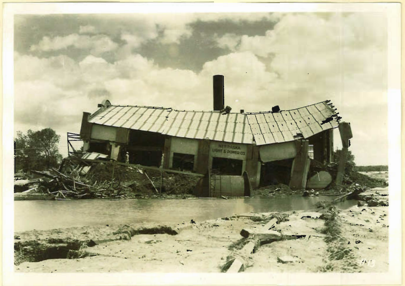
Front view of power plant three days after the flood. Note rails in foreground washed from original location to the right. Debris is being thrown out of the plant Photo by Jaquet
