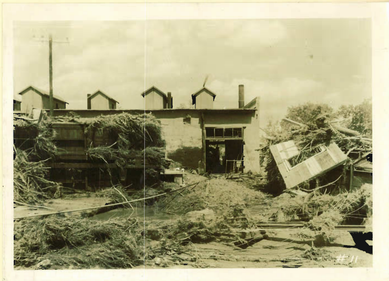
West side of old portion of plant. Note the two cinder cars that were overturned by the water and which later diverted the heavy current from the wall. We spent the larger part of our time on this roof while marooned
