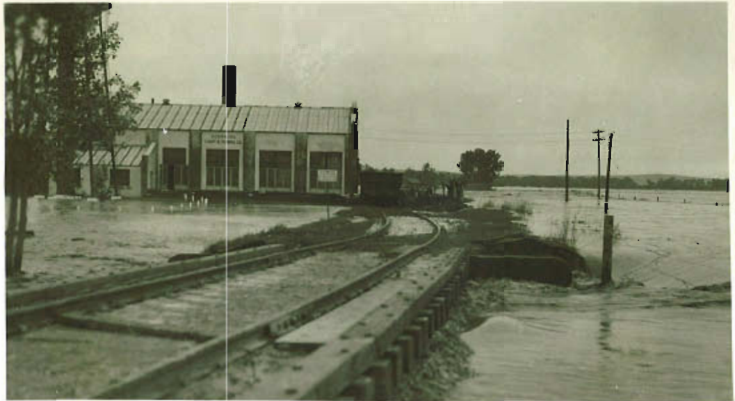
10:00 A.M., a few minutes later the water covered the embankment in the center ground Photo by Geo. Kearns
