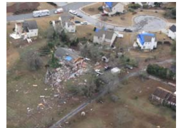
Damage from an EF2 tornado in Buford, GA on 30 November 2010.
