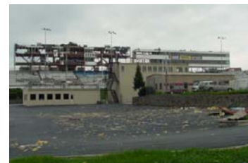
F2 tornado damage at the Atlanta Motor Speedway in Hampton as the remnants of Tropical Storm Cindy moved through Georgia. Damage costs to the AMS alone were over $10 million.
