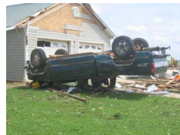
Vehicle destroyed and home severely damaged in Carroll County where a fatality occurred due to a Katrina-spawned F2 tornado.
