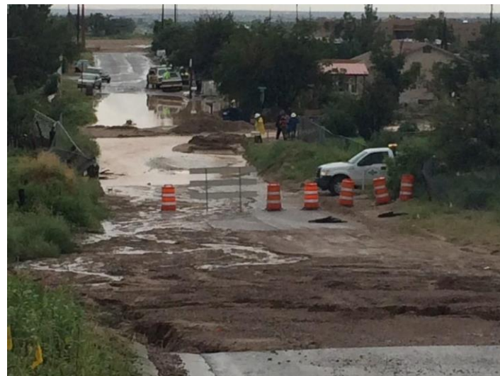
Heavy rains flooded La Union NM on September 17.
