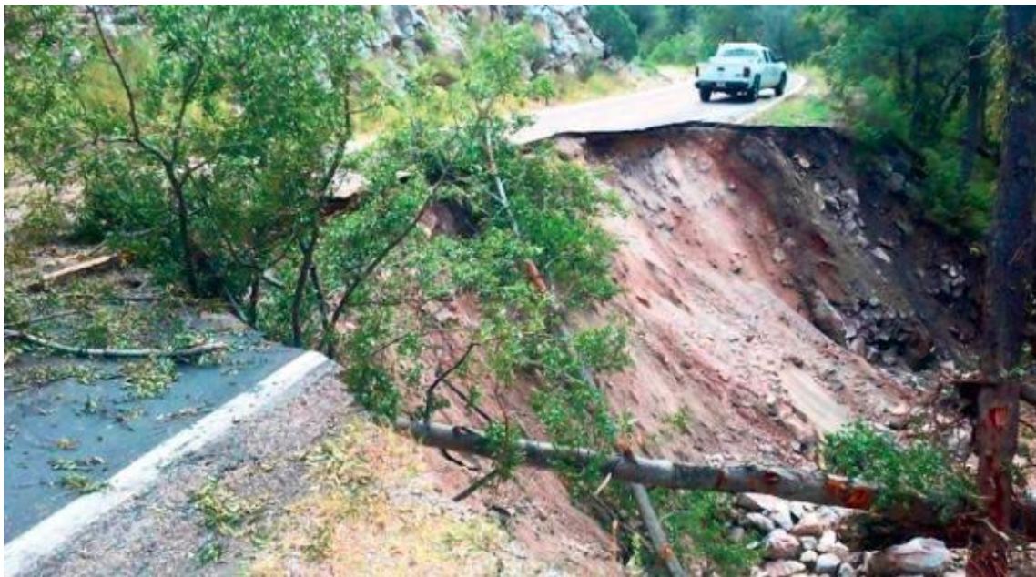
Heavy rains washed out Highway 152 in Sierra County on September 12. (The Herald of Truth or Consequences)
