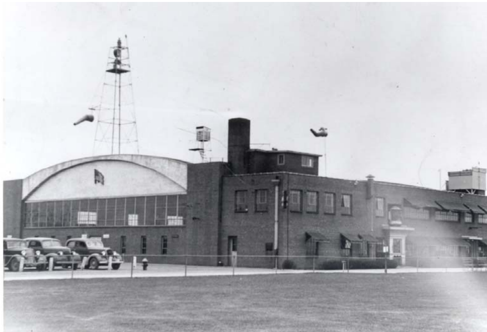
Figure 11. The Des Moines, Iowa, Municipal Airport Hangar, circa 1930's. View is looking southeast. Source: State Historical Society of Iowa.
