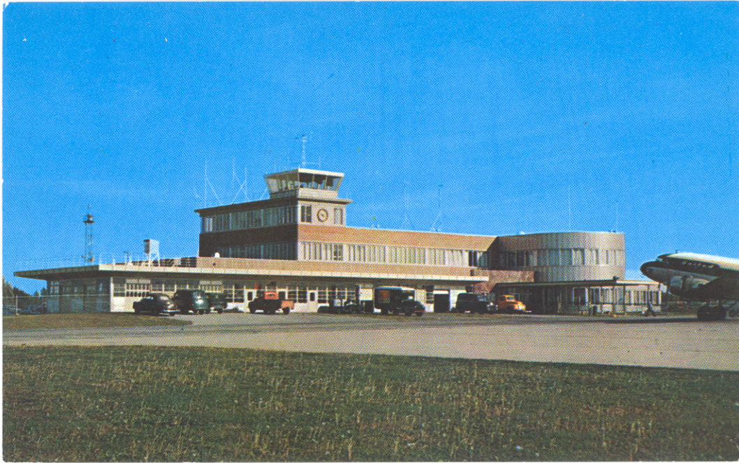
Figure 13. The Terminal Building at the Municipal Airport in Des Moines, Iowa, circa 1952. View is looking southeast. The instrument shelter can be clearly seen mounted on the north roof and the wind instruments on the roof of the control tower.
