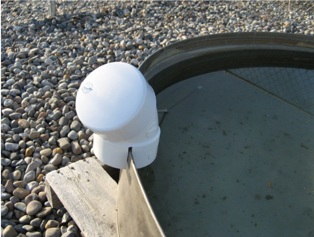
Figure B-8: Street-Elbow Pipe Fitting with Pipe Cap Cover
