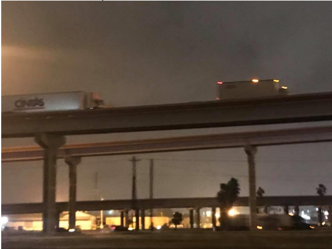
Figure 1. Stranded tractor trailers and other vehicles on glazed overpasses for IH-2 and IH-69E junction in Harlingen, Texas, at around 7 PM CST, January 16 th , 2018.
