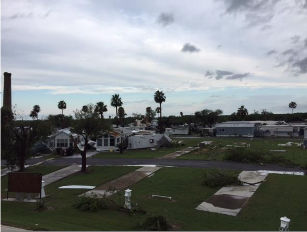
Widespread wind damage to Chimney Park mobile home/RV community south of Mission, Texas, after May 31 st downburst.
