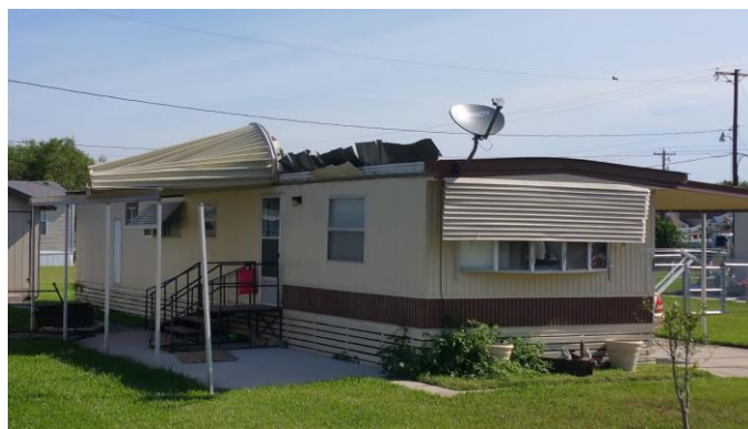
Above: Damage/peel back to a tin roof at the Sun Valley Acres Retirement Park, just north of Interstate 2 in west Harlingen, from wind gusts near 60 mph after midnight on April 19 th . Photo courtesy of Facebook via Dan Joseph at KGBT-CBS Channel 4.
