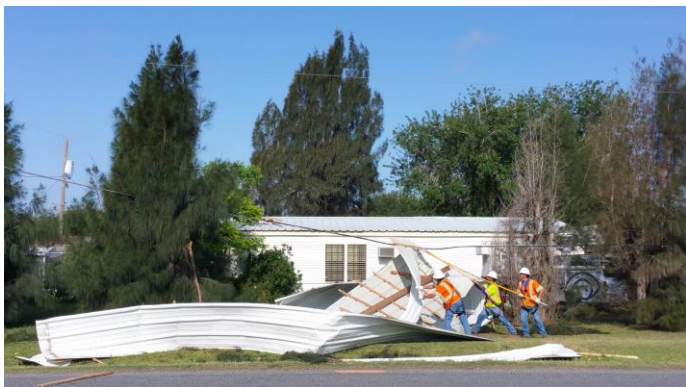
Above: Damage/peel back to a tin roof at the Sun Valley Acres Retirement Park, just north of Interstate 2 in west Harlingen, from wind gusts near 60 mph after midnight on April 19 th . Photo courtesy of Facebook via Dan Joseph at KGBT-CBS Channel 4.
