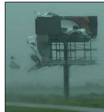
Above: Wind damage to a billboard from Hurricane Lili in October 2002.
